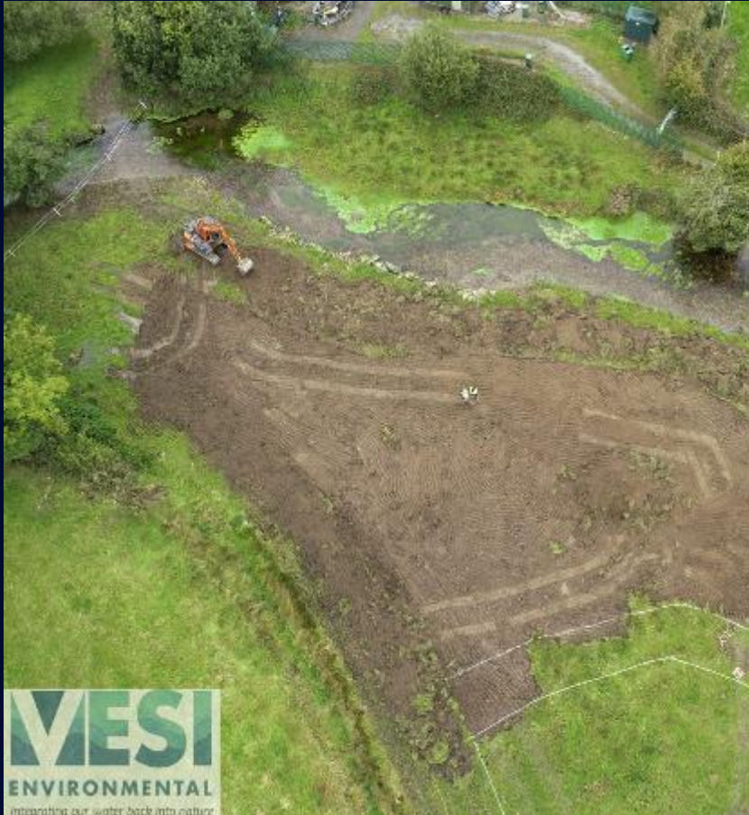
General Site Clearance Completed
