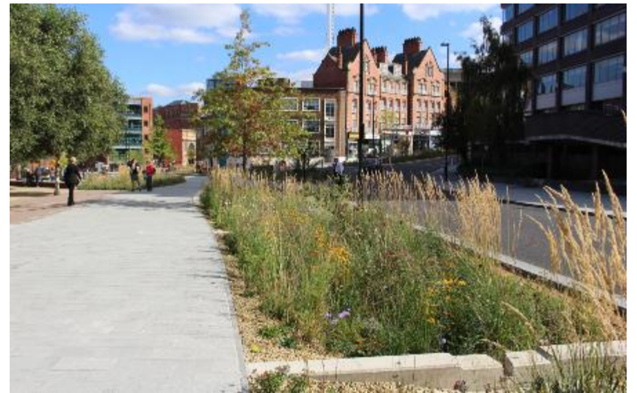
Roadside bioretention raingarden Storing and treating rainfall runoff from road
