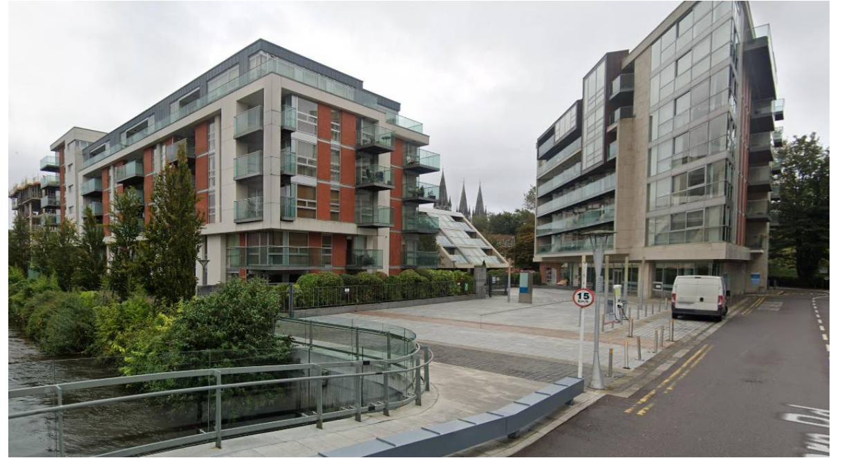
Lancaster Gate, Cork (Clúid Housing)
